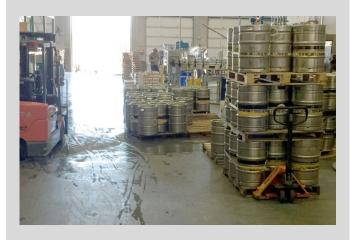
Flowfresh HF is a highly durable, trowel applied cementitious mortar that is installed at thicknesses up to 3/8". Designed for the most arduous of food manufacturing environments the system offers clients an excellent chemical resistance profile combined with temperature resistance up to 250°F intermittently – ideal for environments subject to high temperature processes and hot water washdowns.
