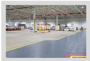
For the spaces that would be faced with more challenging demands, 40,000 square feet of the highly durable epoxy floor mortar <u>Flowtex</u> (1/4") was installed. This system has enhanced abrasion, wear, scratch and chemical resistance, making it suitable for even the most heavy-duty processing environments.
