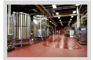
12,000 sq ft of Flowcrete's cementitious urethane floor system, Flowfresh SRQ was installed in a custom blend kitchen-red color within the main production and bottling area thanks to its antimicrobial, chemical resistant and hard-wearing properties.
