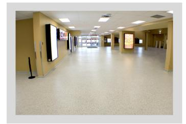
movements in the suspended slab. Combining Flowcretes' decorative, self-level and fast-cure Flowfast Flakes system, installed at 1/8", with a semi-flexible urethane body coat and semi-flexible top coat, the new system has performed incredibly well to date with not one single crack telegraphing through.
